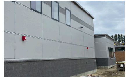
Above: Exterior finishes
